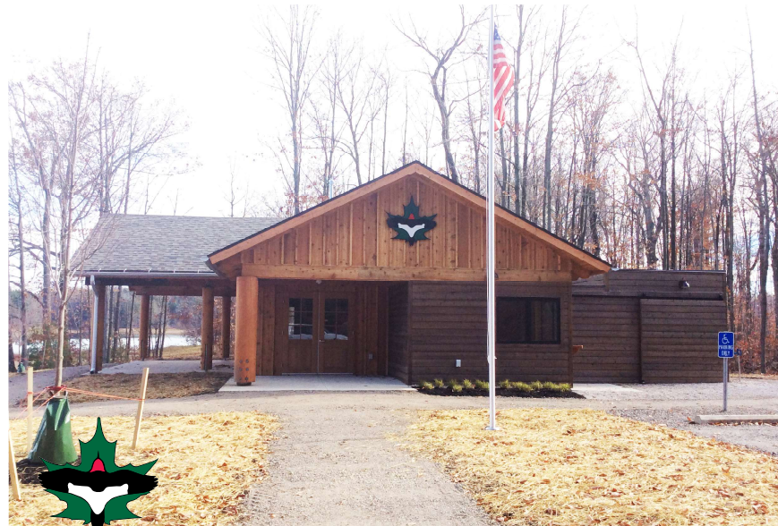
GEAUGA PARK HEADWATERS PARK - BOAT HOUSE 2015
